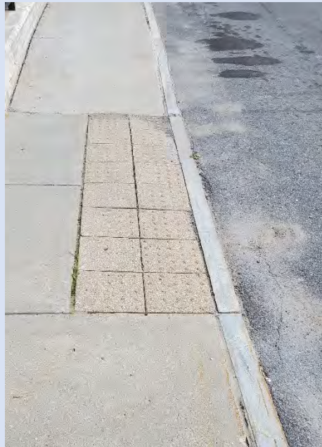
DWS Color Does NOT Contrast from Curb Ramp
