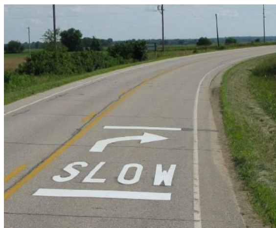
Above, left: "CURVE AHEAD" paired with transverse rumble strips. Right: "SLOW" and arrow.
