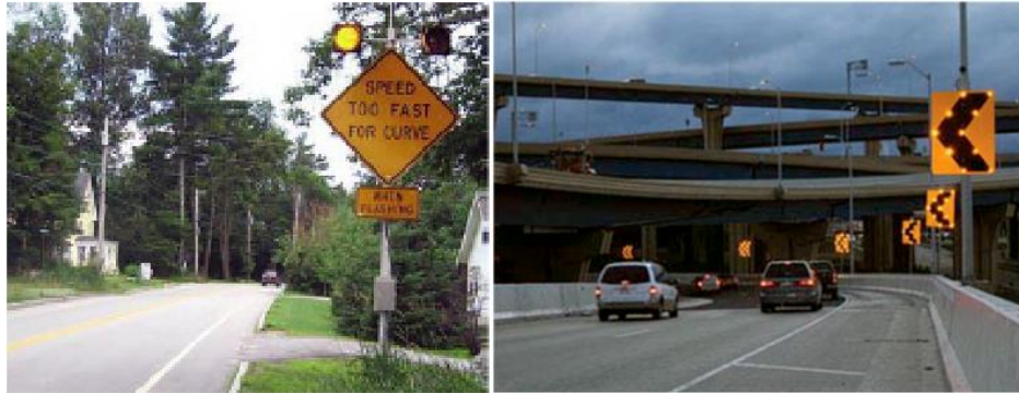
Above, left: "SPEED TOO FAST FOR CURVE" with radar-activated flashing beacons. Right: Sequential Dynamic Curve Warning System with LEDs within chevrons.
