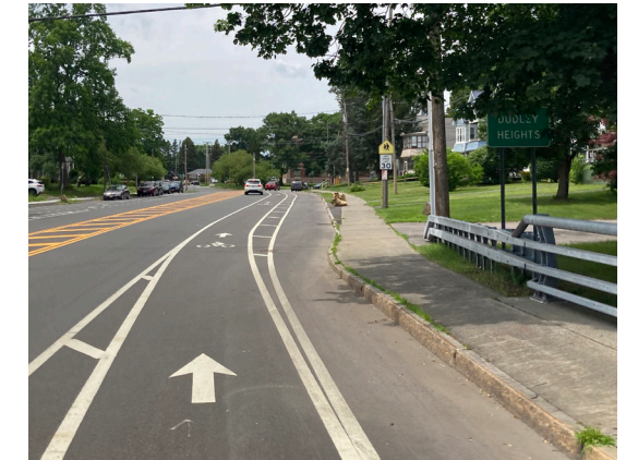
▲ Existing Condition: Northern Boulevard looking west
