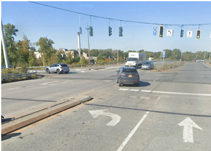
▲ Existing Conditions on Everett Road Bridge
