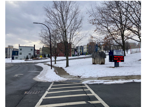
▲ Existing Condition: Lark Drive adjacent to Arbor Hill Elementary School
