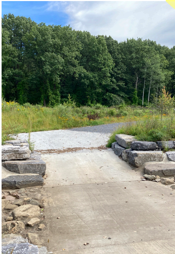
▲ Patroon Creek Spillway in Tivoli Lake Preserve. This area allows the creek to overflow during large storm events.
