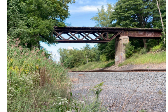
▲ Existing Condition (Abandoned Rail Trestle)
