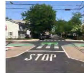
Enhanced pavement markings
