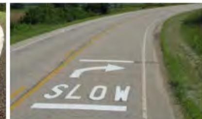
Curve warning pavement markings
